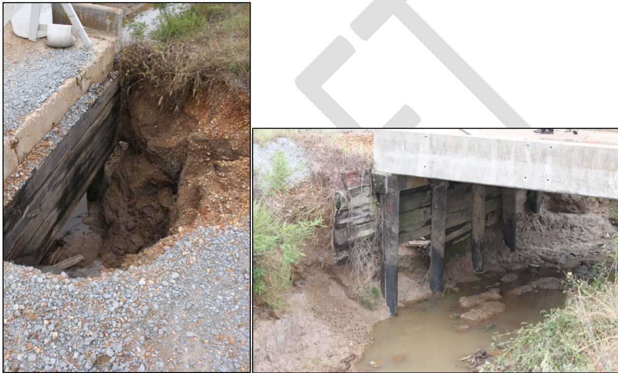
Figure 18: Infrastructure Damage from Channel Erosion
