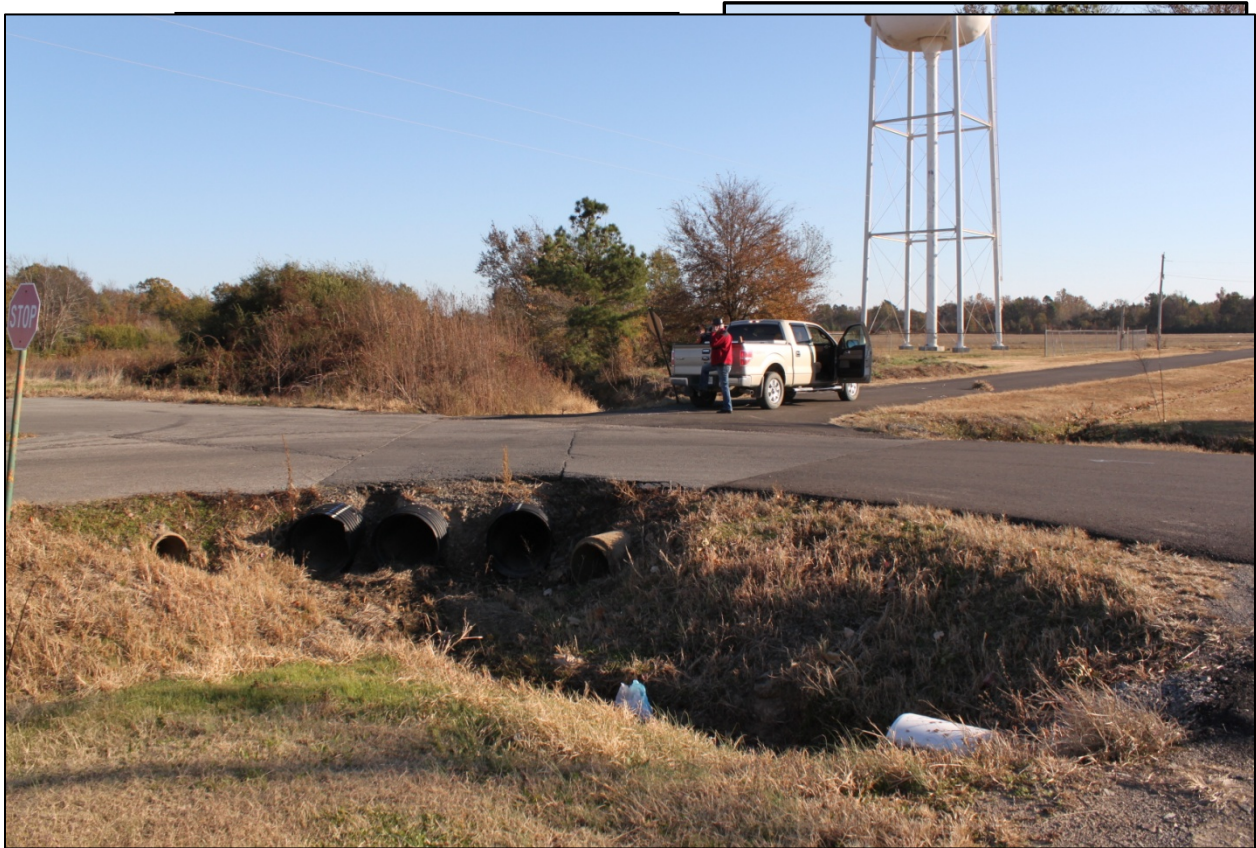
Figure 20. Drainage outlet - Southeast portion of City of McCrory - looking toward Bayou DeView
