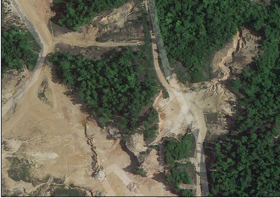
Figure 17e: Typical Gully Sediment Sources: Industrial Source Site
