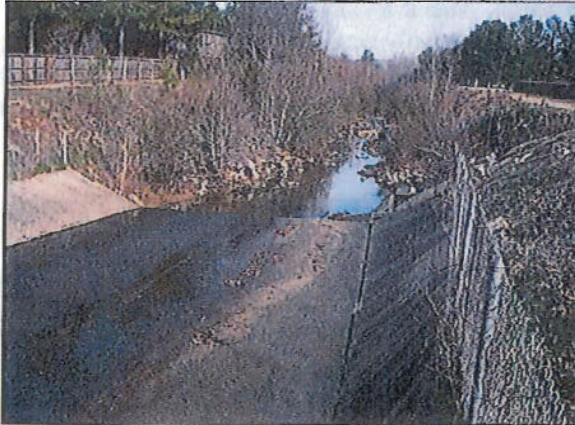
Scour Hole and Bank Erosion at downstream end of Concrete Apron
