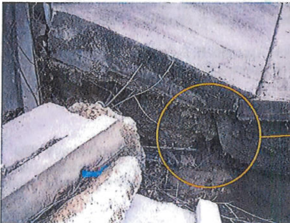
Undermining at left bank ascending wing wall..
