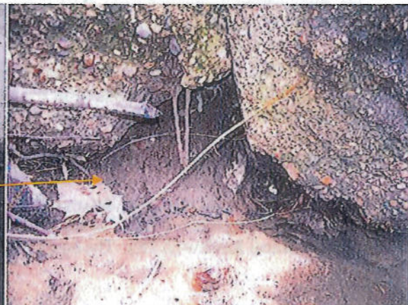
Detail of the Undermining
