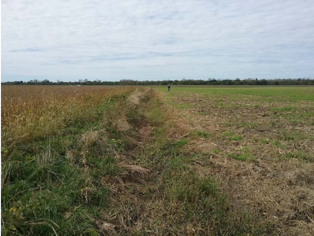
Figure 7. Existing condition of ditch proposed to be modified to facilitate seepwater drainage at the Below Charleston Mile 24 project area, Mississippi County, Missouri.
