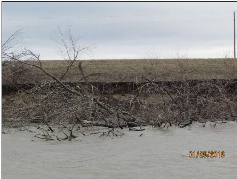
Figure D.5 – Stream bank erosion looking east from chute
