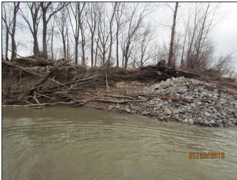
Figure D.6 – Stream bank erosion end of existing riprap revetment
