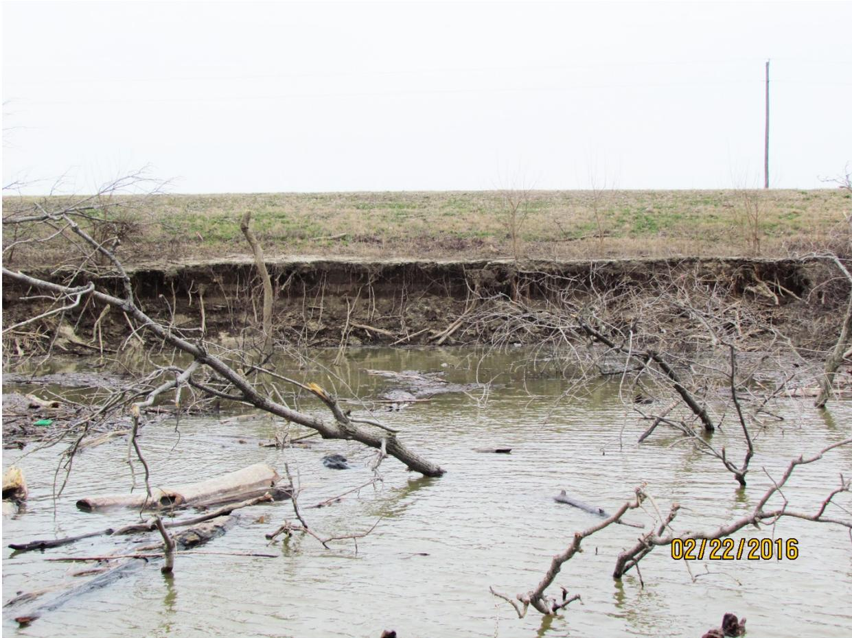
Figure 2. Photograph of the active scour occurring at the Dyer County Little Levee PL 84-99 Project Area, in Northwestern Tennessee.
