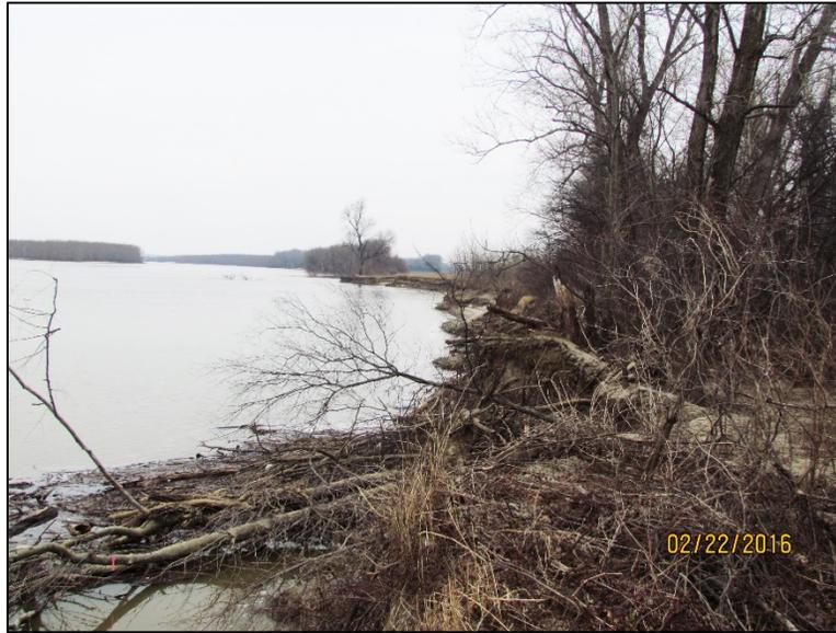
Figure D.3 – Stream bank erosion looking north from end of existing riprap
