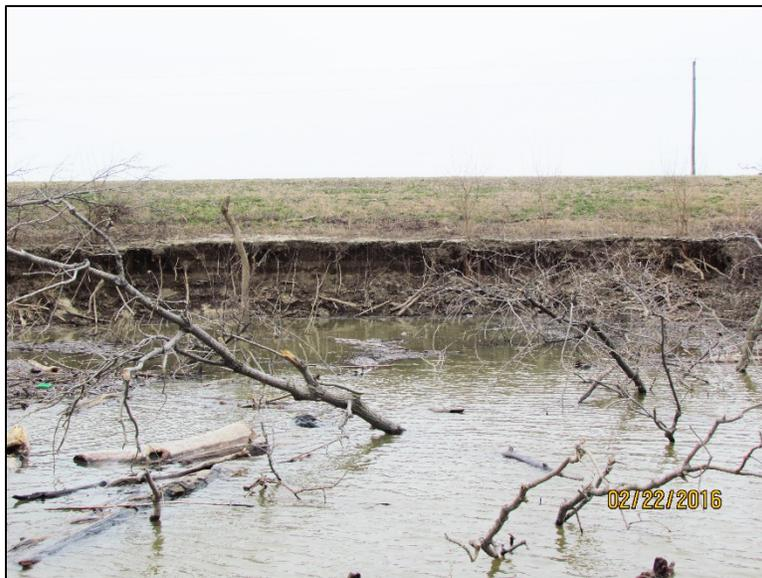
Figure D.2 – Stream bank erosion looking east from the chute
