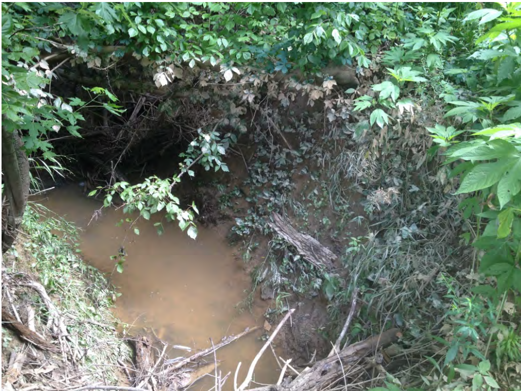
Photo 4: A view of the central drain across the existing access road at the culvert. The culvert will be removed at this location and the drain will be plugged.
