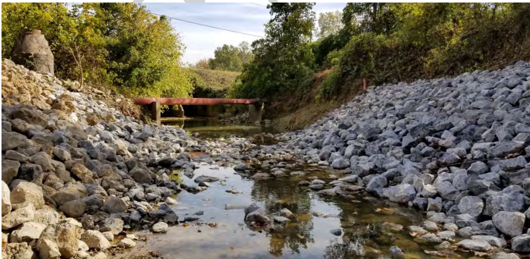
Figure 31. Nolehoe Creek riprap structure immediately upstream of Pleasant Hill Road Culvert
