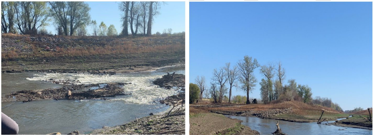
Figure 4. Existing project area scour conditions (left) and left descending bank (right), St. Johns Bayou Outlet Ditch Repair Project (Phase 1), New Madrid County, Missouri.
