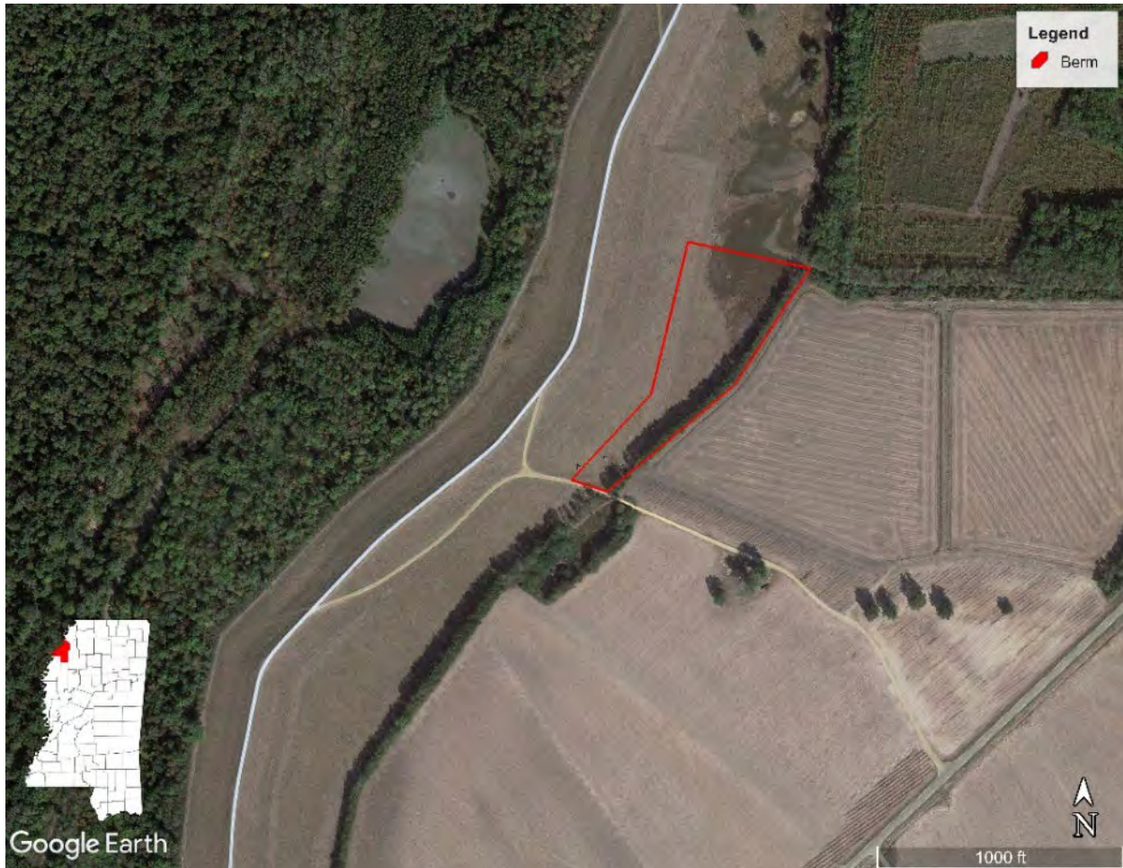
Figure 3. Aerial of site conditions at the proposed northern seepage control berm along the Mississippi River mainline levee at the Sherard project area, Coahoma County, Mississippi.
