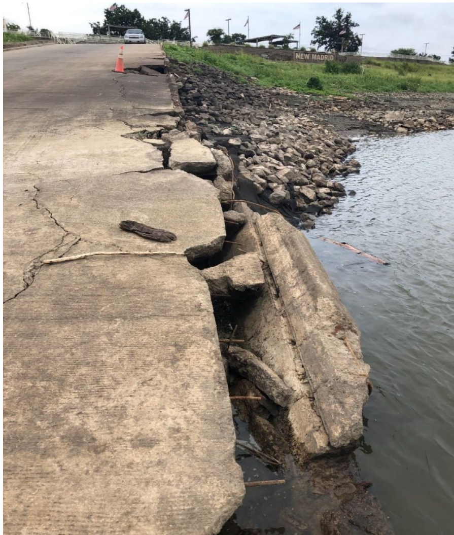
Figure 2: Concrete damage and scour conditions at the New Madrid boat ramp, New Madrid County, Missouri.
