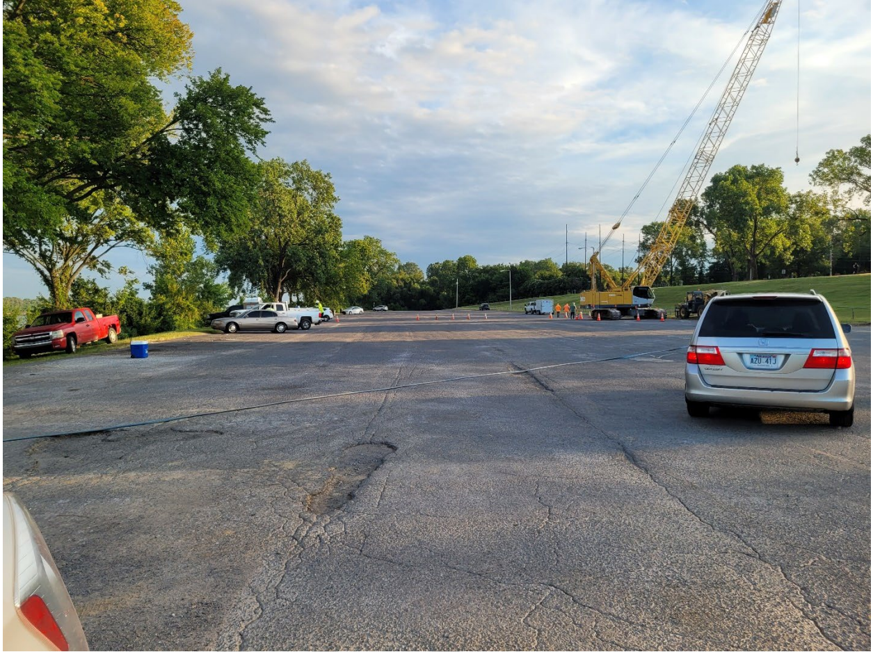
Figure 6: Existing parking lot, showing potholes and cracks in asphalt. Facing north, from south end of project area.
