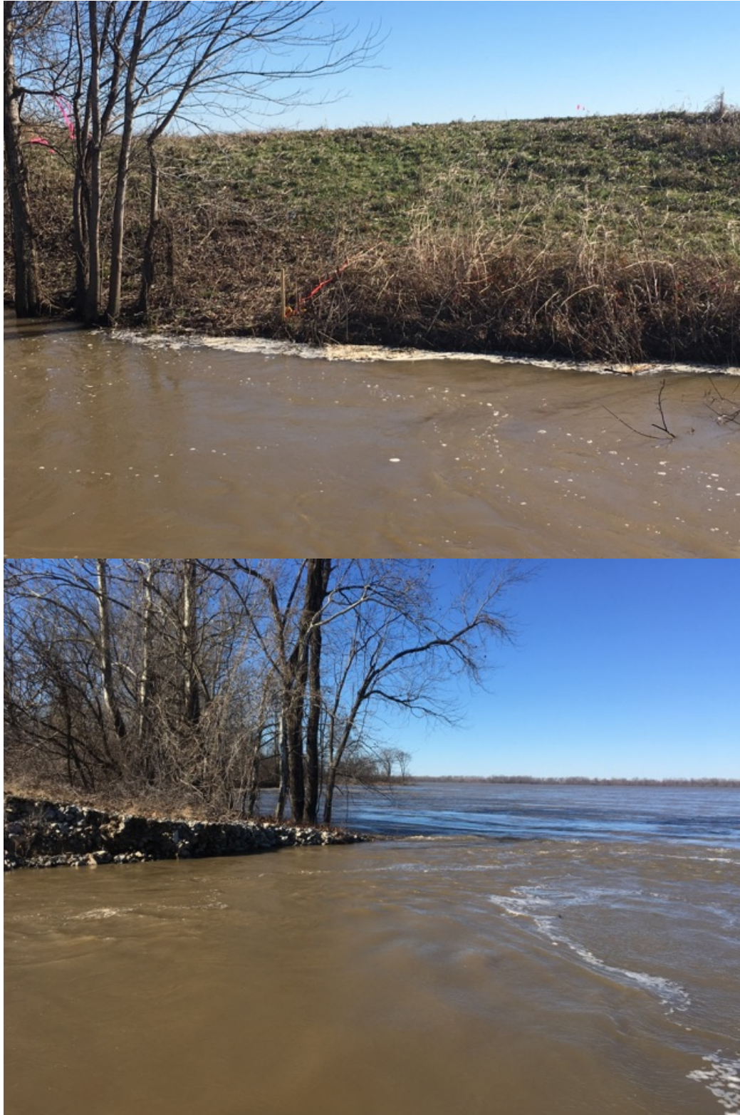
Figure 2. Photographs of the active scour that prompted the emergency repairs at the Dyer County Little Project Area, in Northwestern Tennessee.
