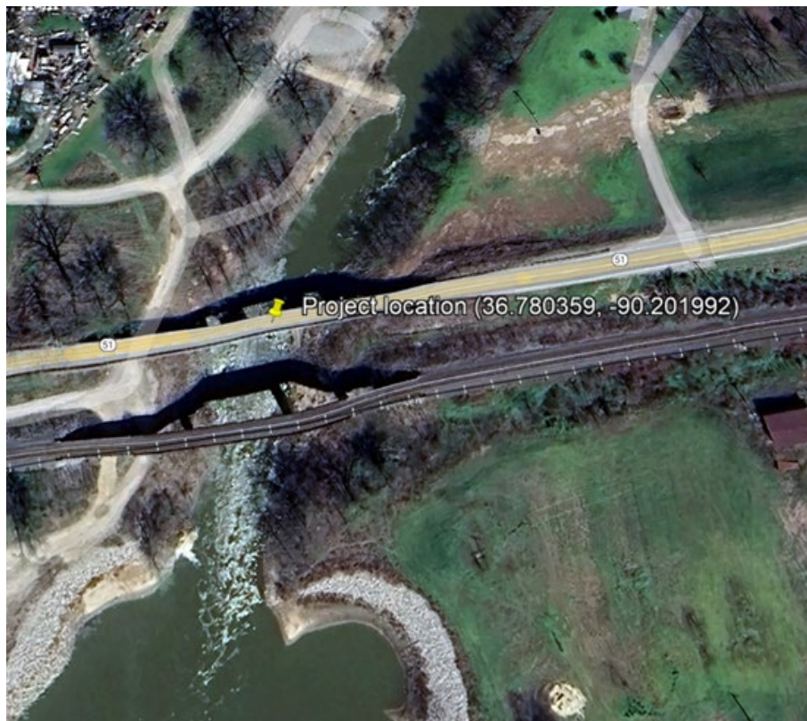
Figure 1. Location of proposed bridge removal and replacement in Butler County, MO.
