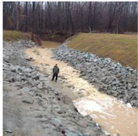
Figure 12. Rock Chute structure on a similar stream in West Tennessee.
