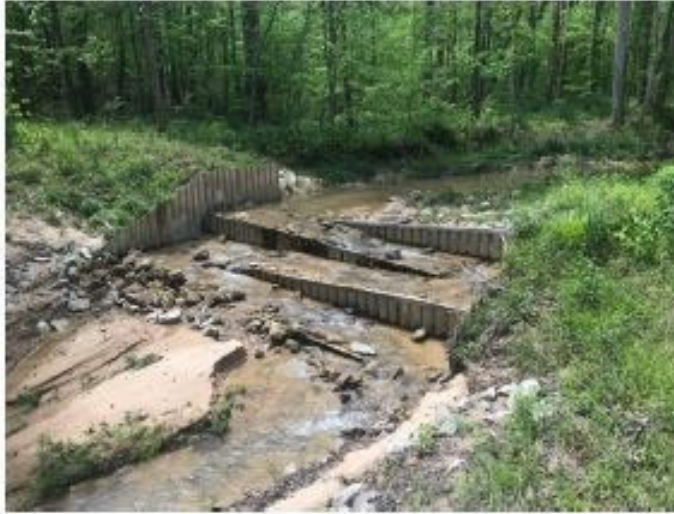
Figure 11. Fish Passage Structure in Upper Piney Creek.
