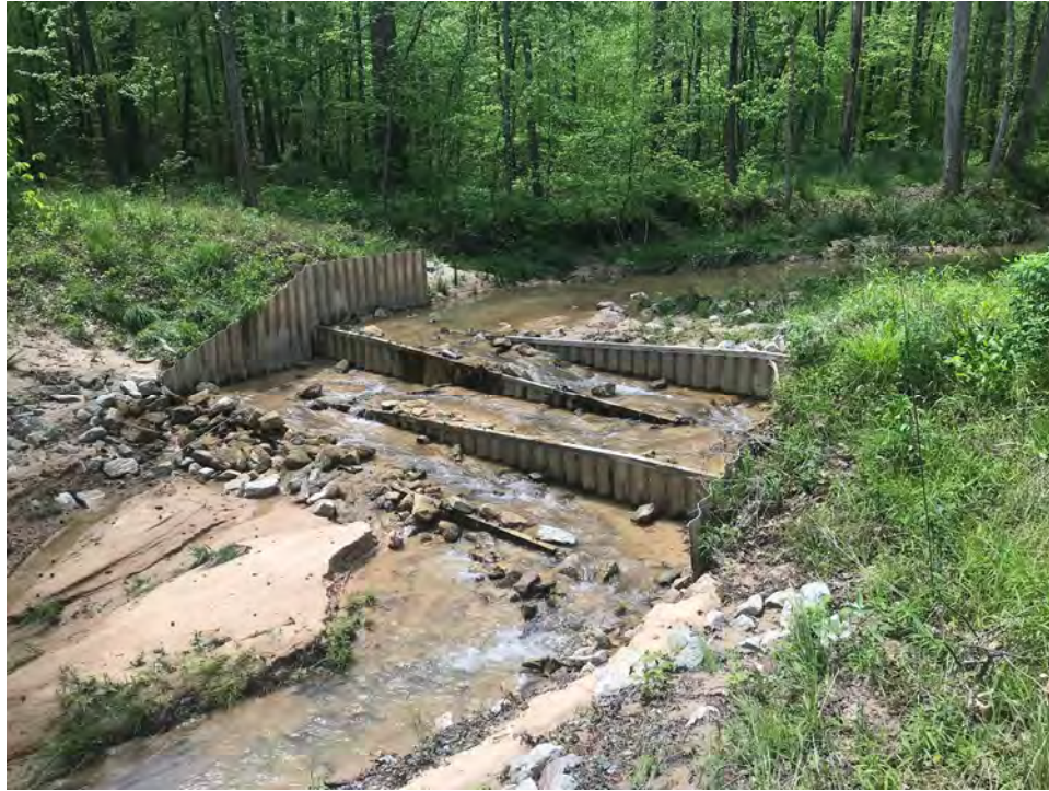
Figure 4 - Minor Grade Control / Fish Passage Example
