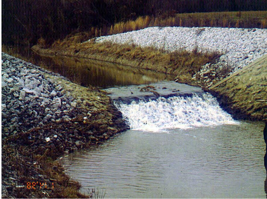
Figure 13. Long Creek-Low Drop Grade Control Structure
