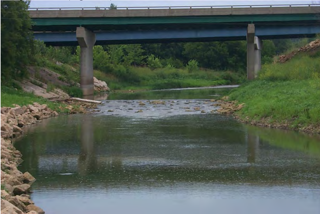
Figure 15. Sinsinawa River, Northern Illinois; Loose Rock Riffle Grade Control with downstream right bank LPSTP, notice floodplain bench forming upstream of bridge
