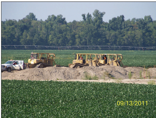
Harvesting sand from the surrounding land at the center crevasse Tuesday. Crews were mobilized here to begin preparing the ground for construction.
