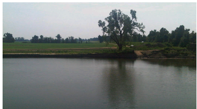
Center crevasse near Seven Island Conservation Area. The existing levee is visible behind the tree.
