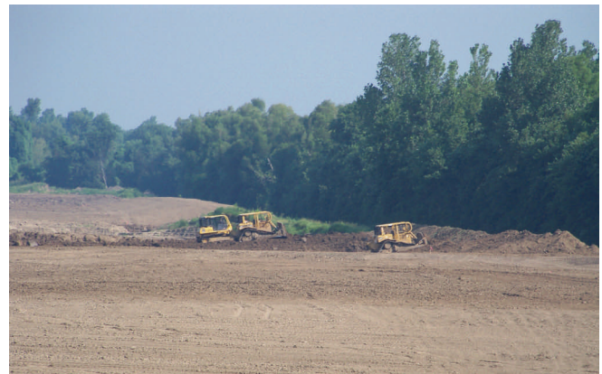
Repairing the levee at the upper crevasse.
