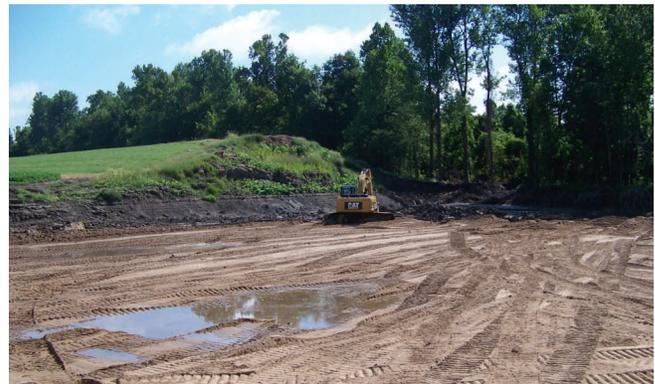
**Sand is used to fill the scour holds near Birds Point. Clay will later be used to cap the hole.**
