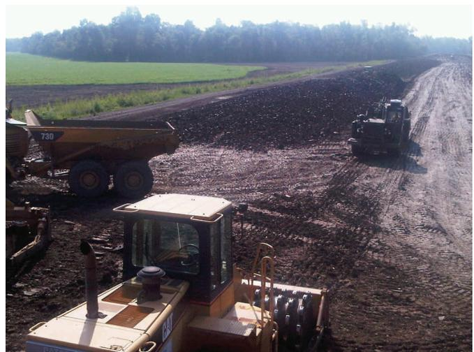
**A Vicksburg-based crew removes excess water in the soil at the lower crevasse. Once at the proper moisture content, the material will be compacted into the levee.**
