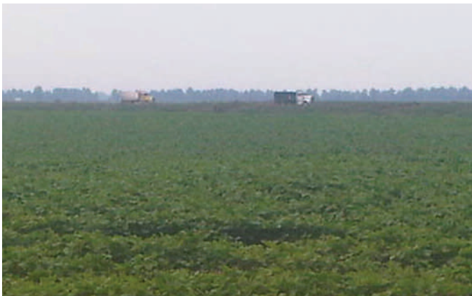
Dump trucks leave the site after delivering sand at the upper crevasse. More than 58,000 tons of sand has been delivered to date.
