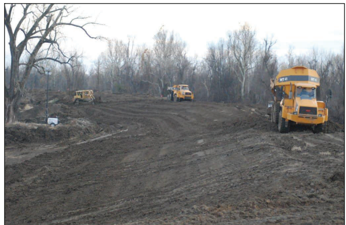
Crews reconstruct the levee at the center crevasse Dec. 3.
