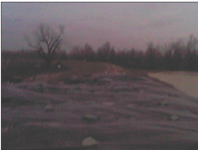
Water creeps up the toe of the levee at the center crevasse Monday evening (river is on right side). The forecasted crest is expected to put about five feet of water on the 15-foot-high levee.
