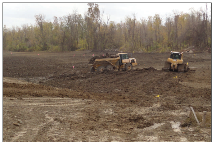
Crews deliver and spread clay Sunday at the center crevasse.
