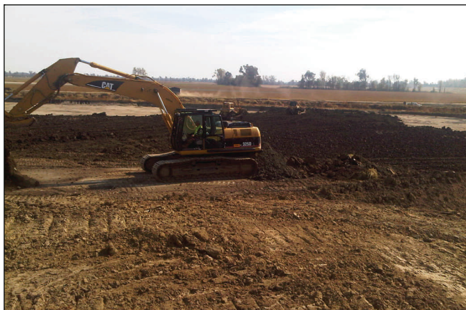
Crews spread and compact clay at the center crevasse Wednesday. The excavator is removing asphalt.
