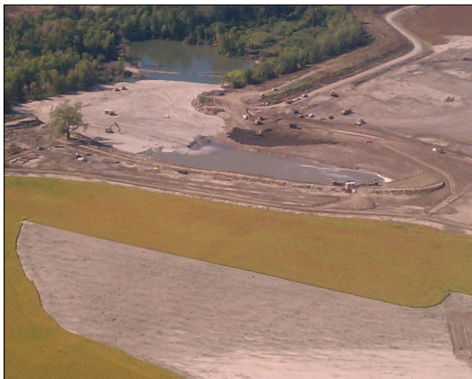
The center crevasse scour hole as seen from the air Oct. 25 during dredging. The area to the right of the levee was filled in after this photo was taken. (Photo by Brad Hahn, courtesy of Great Lakes Dredge & Dock Company)
