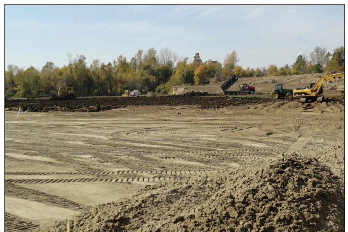
The scour hole at the center crevasse is filled with sand. Dredging ended Monday morning.
