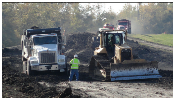
Crews spread clay landside of the levee at the upper crevasse Wednesday.
