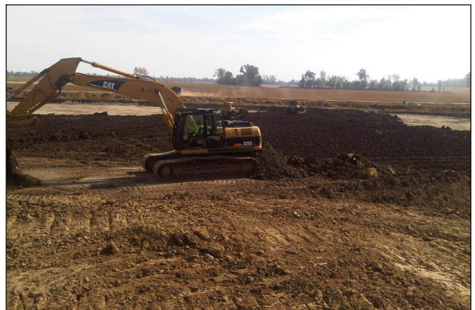
Crews spread and compact clay at the center crevasse Wednesday. The excavator is removing asphalt.
