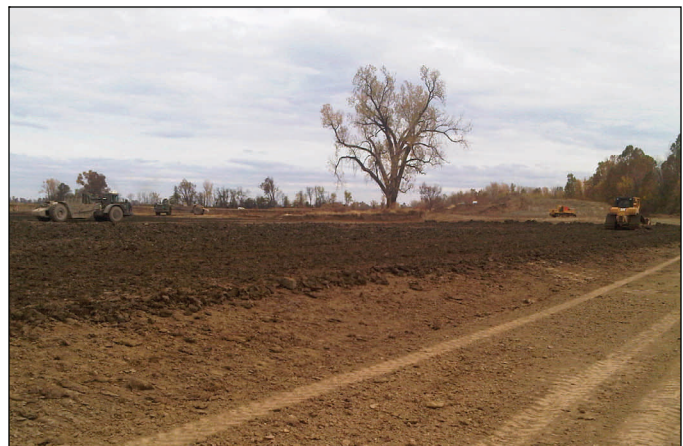
Crews disk and compact clay after it is placed in the scour hole at the center crevasse Tuesday.
