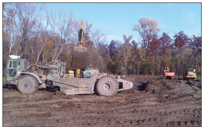
Crews load clay at a newly-acquired borrow site Monday. The clay is bound for the scour hole at the center crevasse.
