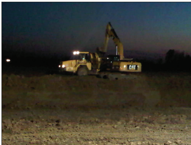
An excavator operator loads an off-road dump truck Monday night with clay that will fill the land-side berm. Each off-road truck can carry up to 25 tons of clay. The District began night operations Saturday.
