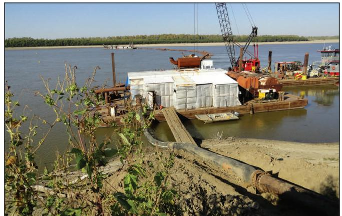
**The dredge (background) pumps sand to a booster pump (on barge, center), to the shore pipeline (foreground), and then to the scour hole at the center crevasse.**
