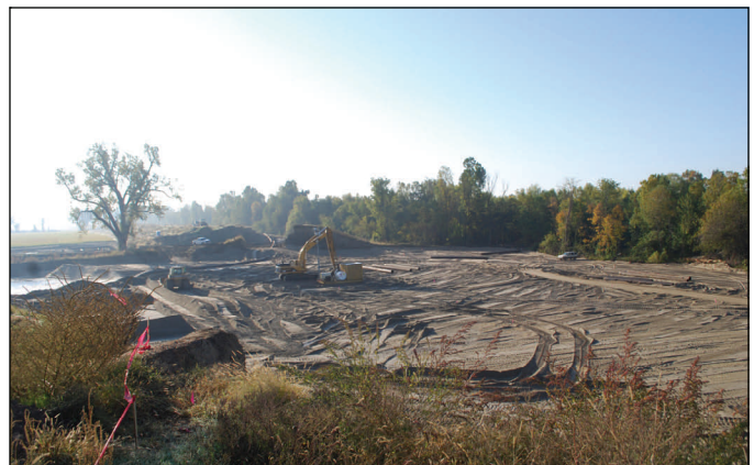
The dredge contractor pumps sand into the scour hole at the center crevasse Sunday.
