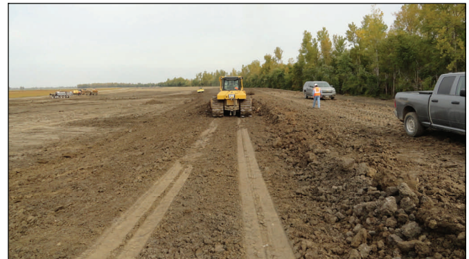
Clay embankment is placed landside of the levee at the upper crevasse Sunday to prevent seepage.
