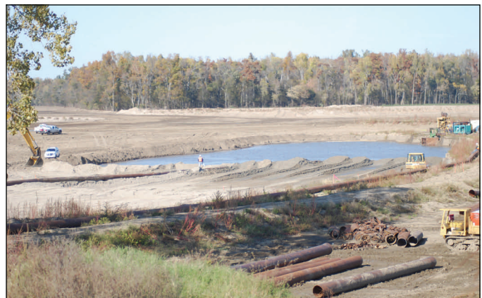
The dredge Iowa pumps sand into the scour hole at the center crevasse Sunday. Dredging ended Monday.
