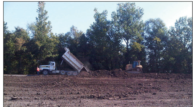
Clay embankment is dumped and placed in the levee at the upper crevasse Wednesday.
