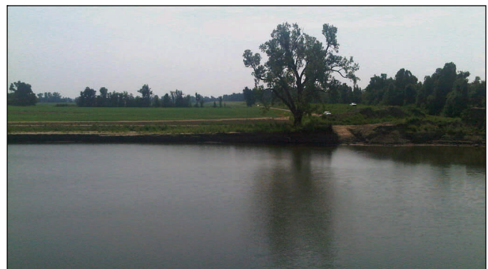
Center crevasse near Seven Island Conservation Area. The existing levee is visible behind the tree.
