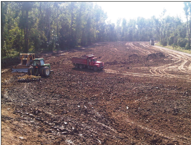
A Vicksburg crew processes material Sept. 21 at the lower crevasse to remove excess water. The soil here is poorly drained and extra effort is required to reduce the moisture content to a workable level. The crew resumed processing material Tuesday.
