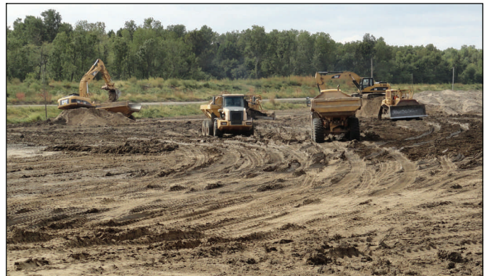
Loading sand at the center crevasse today. The sand is being used to fill the scour hole at the center crevasse.
