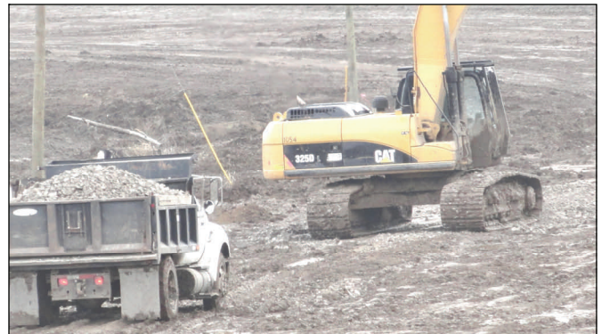
The District's repair team places rock at the center crevasse Feb. 15 to stabilize the roadway.
