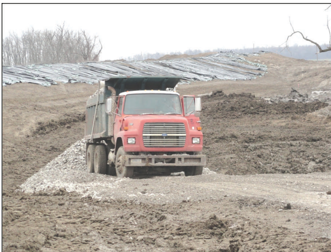
The team performs road maintenance at the center crevasse Feb. 9. Here, the team places rock to stabilize the eastern access road.
