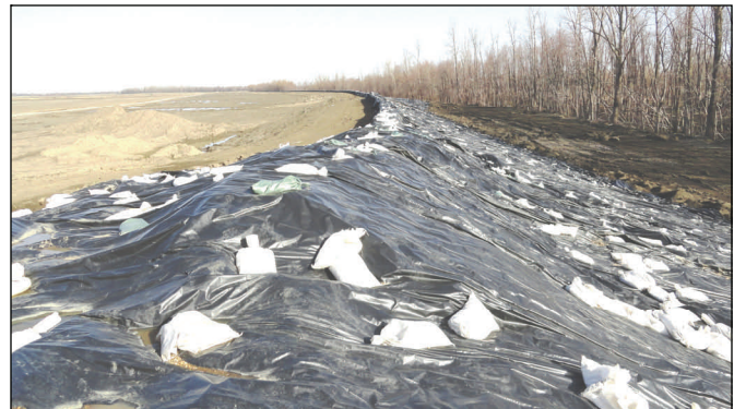
Plastic sheeting to protect the levee and HESCO barriers is shown in this March 1 view.
