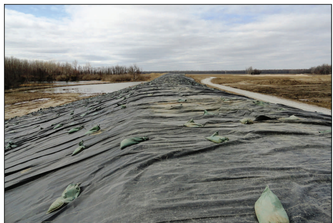
A March 1 view of the repaired levee at the center crevasse. The access road is visible at right.
