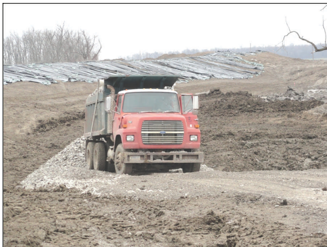
The team performs road maintenance at the center crevasse Thursday. Here, the team places rock to stabilize the eastern access road.
