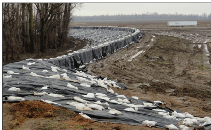
The repair team completed repairs to the plastic at the upper crevasse Feb. 2. The team also added additional sandbags to better hold the plastic in place.
