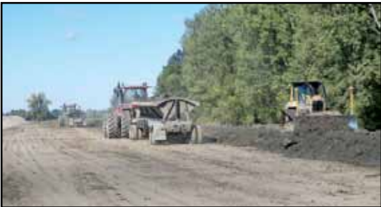
Hydraulic side dump trailers place clay embankment material at the upper crevasse to restore the Birds Point-New Madrid Floodway frontline levee to its full height equivalent to 62.5 feet on the Cairo gage. (USACE photo by Donny Davidson)
