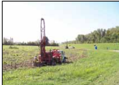
Contractors make pilot hole borings to test the soil before drilling relief wells at Island 8 in Kentucky and Tennessee. (USACE photo by Donny Davidson)
