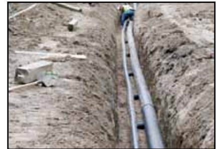
Installing pipes as part of the operating mechanism at the upstream end of the upper levee crevasse. (USACE photo by Donny Davidson)
