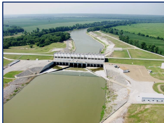
W.G. Huxtable Pumping Station
