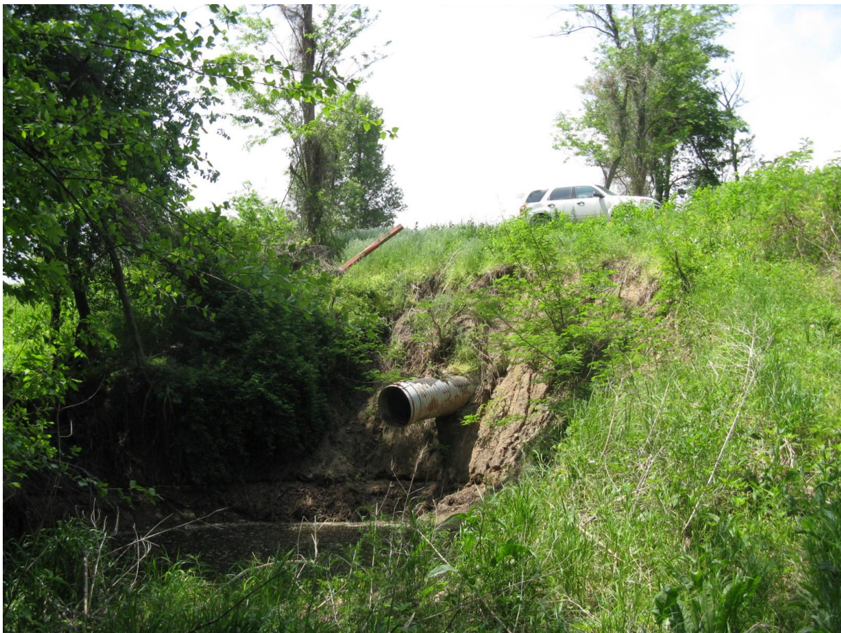
Figure 4. Floodside view of existing culvert pipe and eroded section of the Farrenburg Levee.
