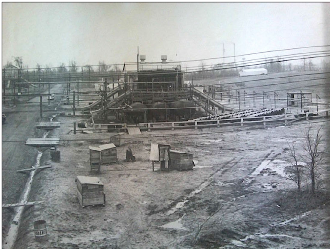
Figure 4-09. Tennessee Powder Company construction ca. 1940 (after Lauderdale 2013a).
