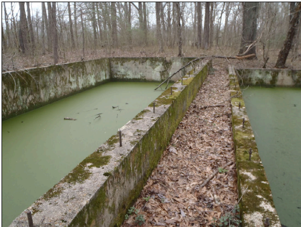
Figure 5-35. Locus L view north from right of stairwell (P2282470).
