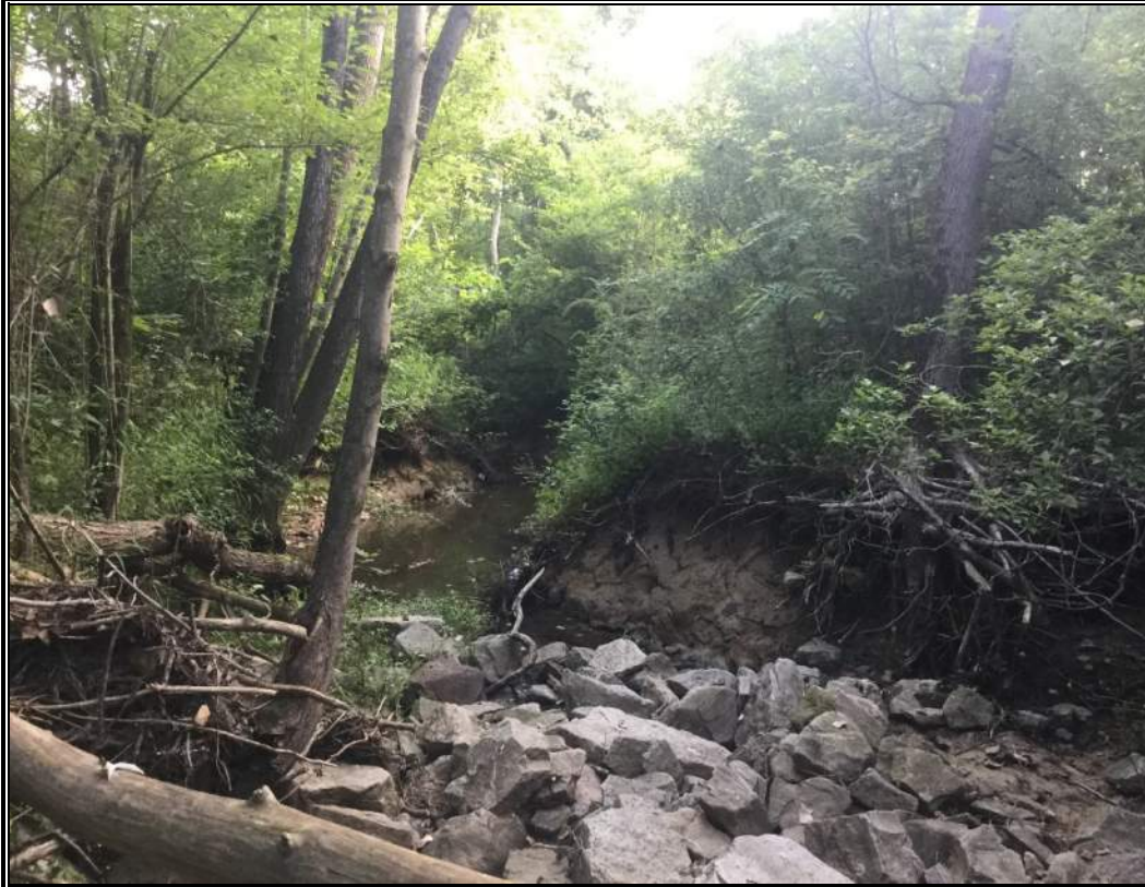
Photo: 83 By: A. Fowler Date: 19 July 2017 Lat/Long: 35.3299, -89.8907 Feature: STR-7
