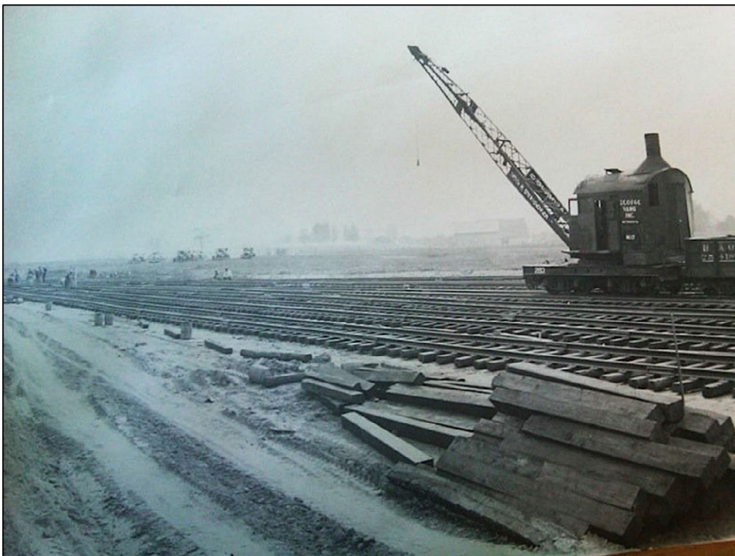
Figure 4-12. Tennessee Powder Company construction ca. 1940 (after Lauderdale 2013a).
