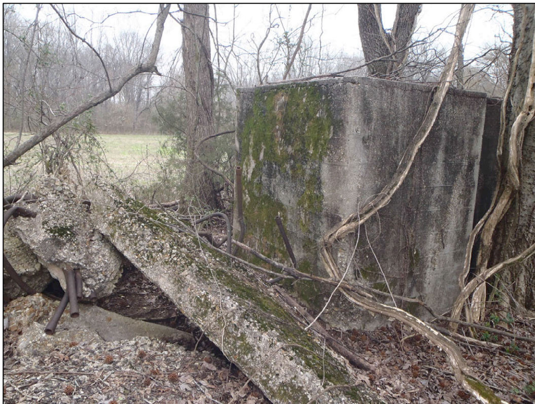
Figure 5-27. Locus F southern portion, view east (P2282447).
