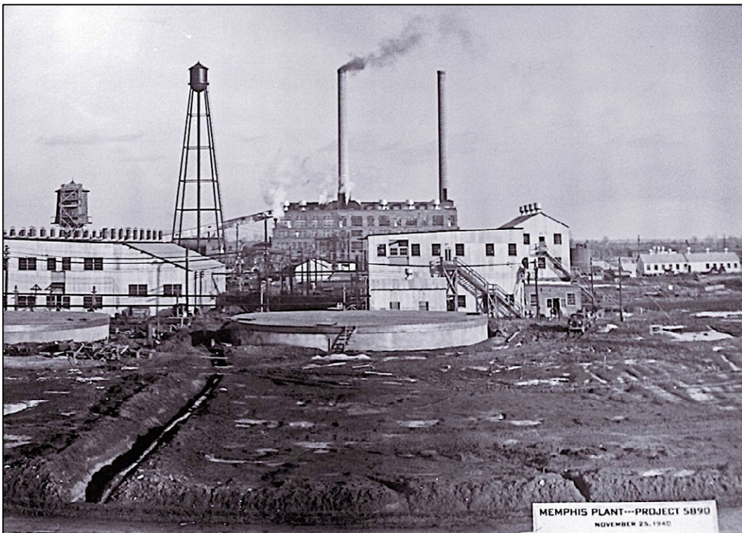
Figure 4-08. Tennessee Powder Company construction ca. 1940 (after Lauderdale 2013b).
