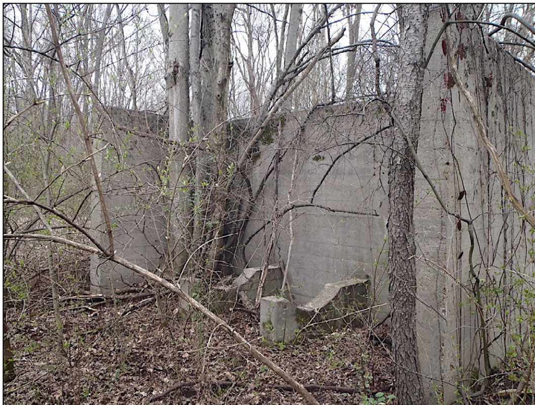
Figure 5-33. Locus J structure interior, view northeast (P2282460).
