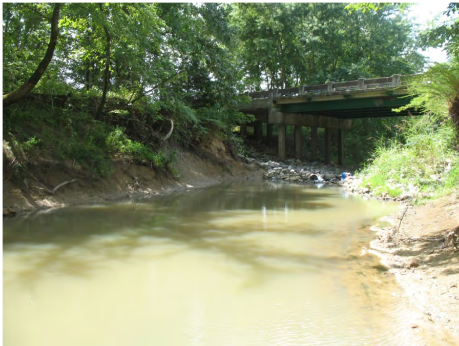
Photo 8: A view of Crooked Creek at the approximate location of the flood control structure near the crossing of Donnell Road. Photo was taken facing downstream (west).
