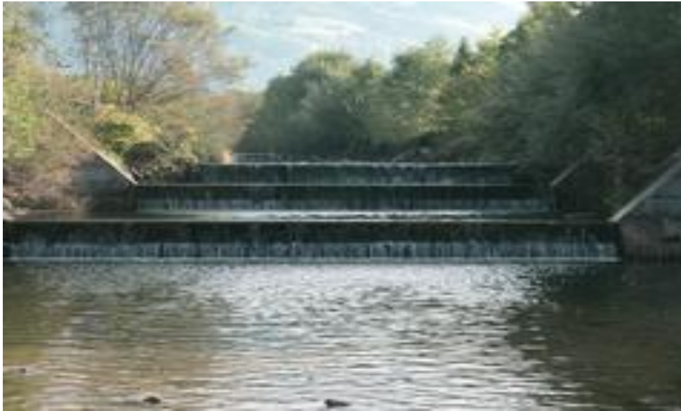
Exhibit 2. Typical Grade Control Structure
