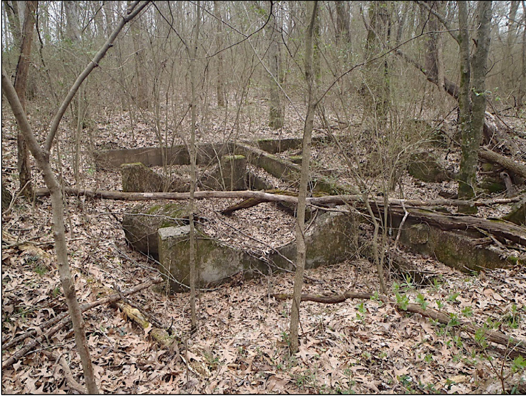
Figure 5-14. Locus A foundation with industrial tank supports, view north (P2282417).
