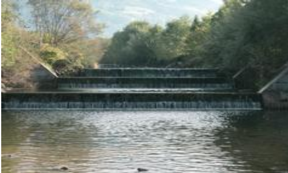
Exhibit 2. Typical Grade Control Structure
