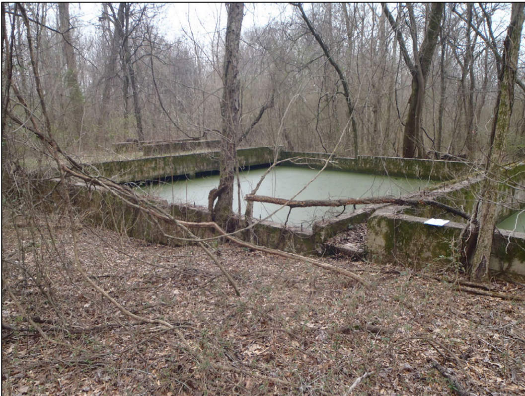
Figure 5-37. Locus L view southwest (P2282472).
