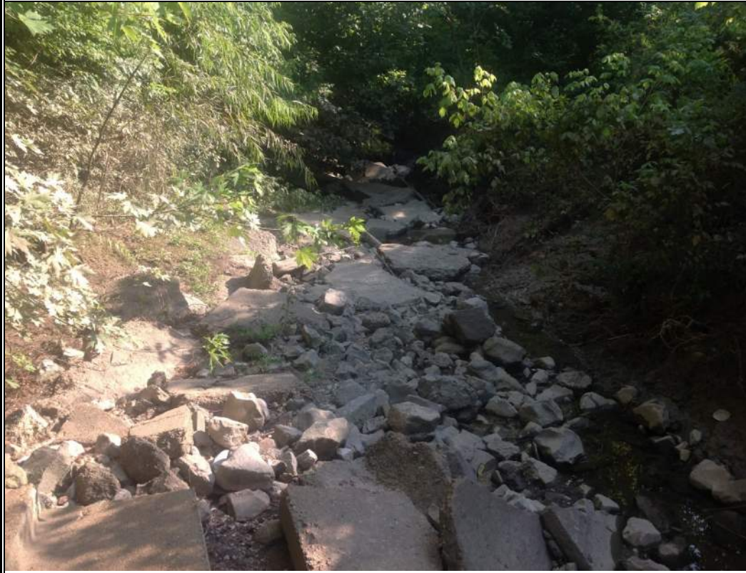
Photo: 77 By: G. Lynch Date: 12 July 2017 Lat/Long: 35.3347, -89.9080 Feature: STR-3
