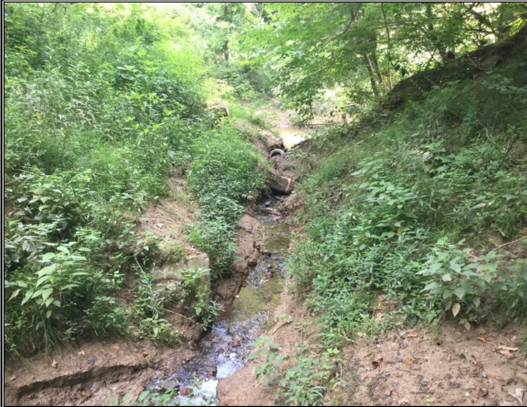
Photo: 91 By: A. Fowler Date: 19 July 2017 Lat/Long: 35.3289, -89.8840 Feature: STR-12
