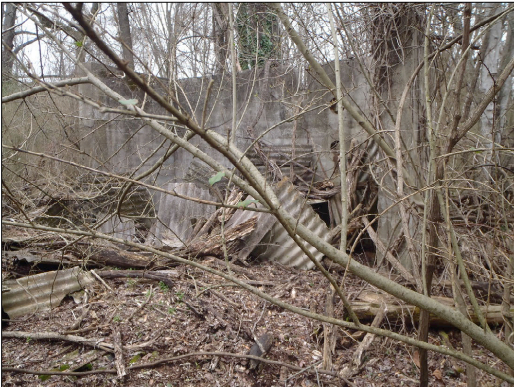
Figure 5-25. Locus E interior of larger structure with corrugated roofing, view northeast (P2282438).
