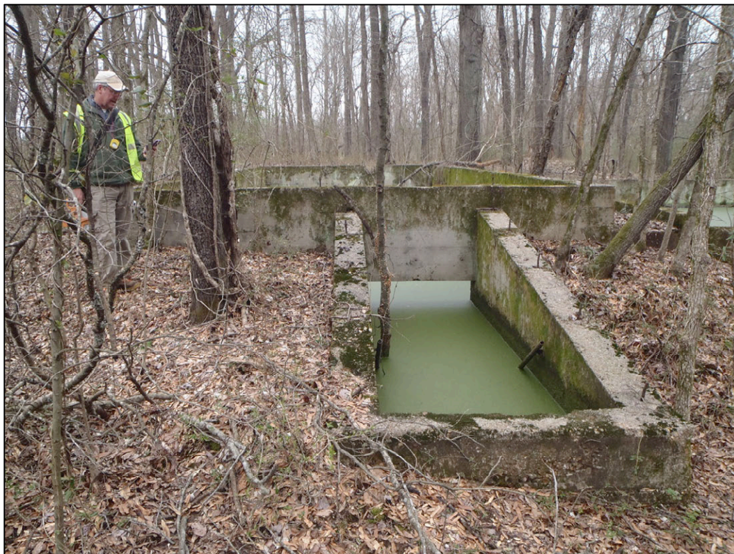
Figure 5-34. Locus L stairwell view north (P2282468).
