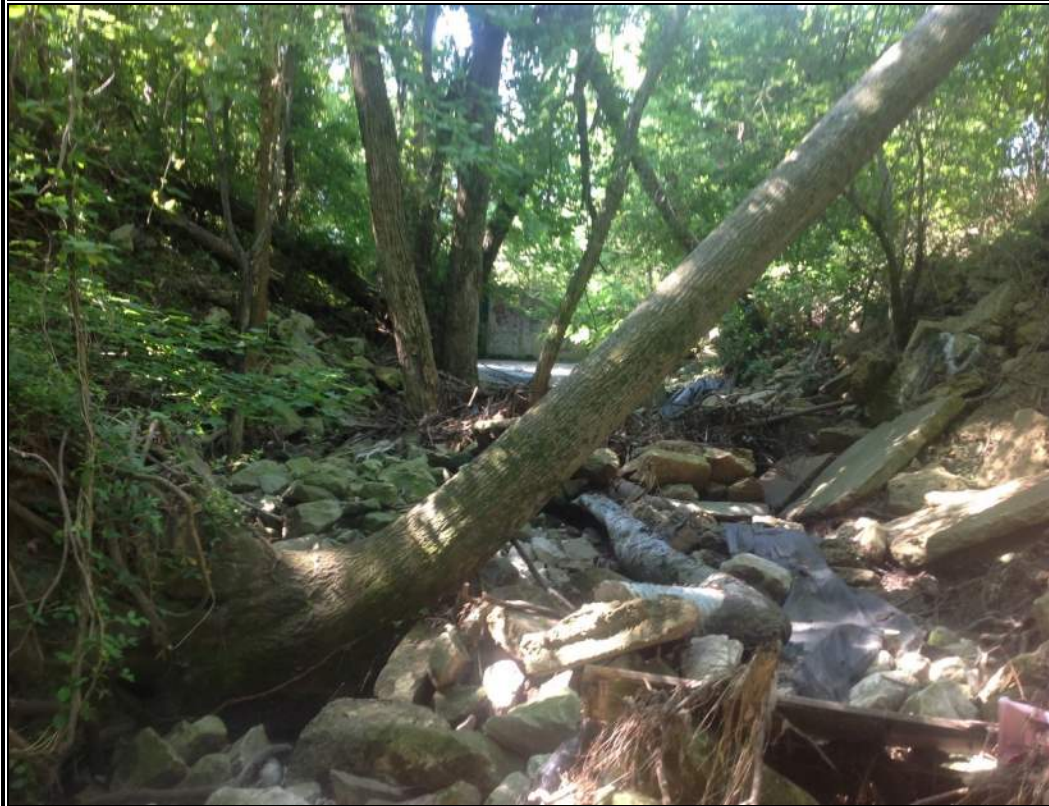
Photo: 80 By: G. Lynch Date: 14 July 2017 Lat/Long: 35.3318, -89.8969 Feature: STR-4
