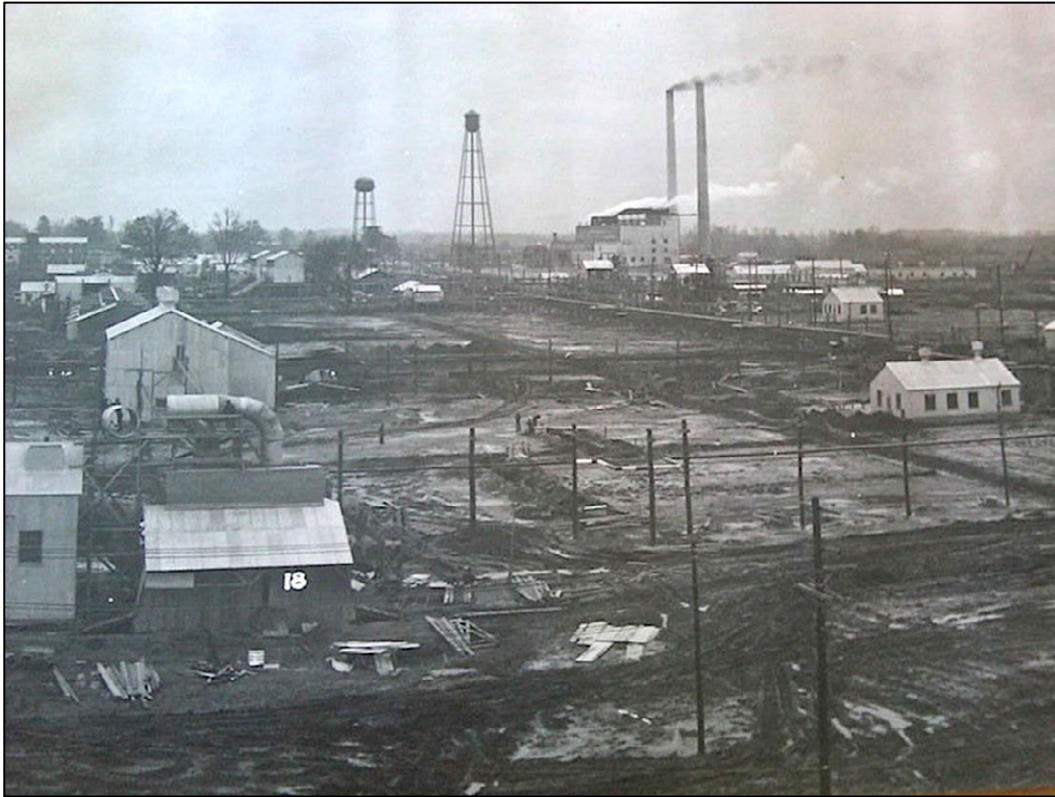
Figure 4-07. Tennessee Powder Company construction ca. 1940 (after Lauderdale 2013a).
